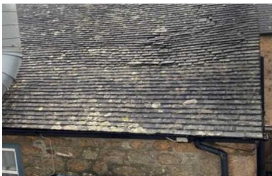
Fig. 7: The north-west elevation of the south wing of Kavorna, showing slate rippling, with details of traditional vernacular construction.
