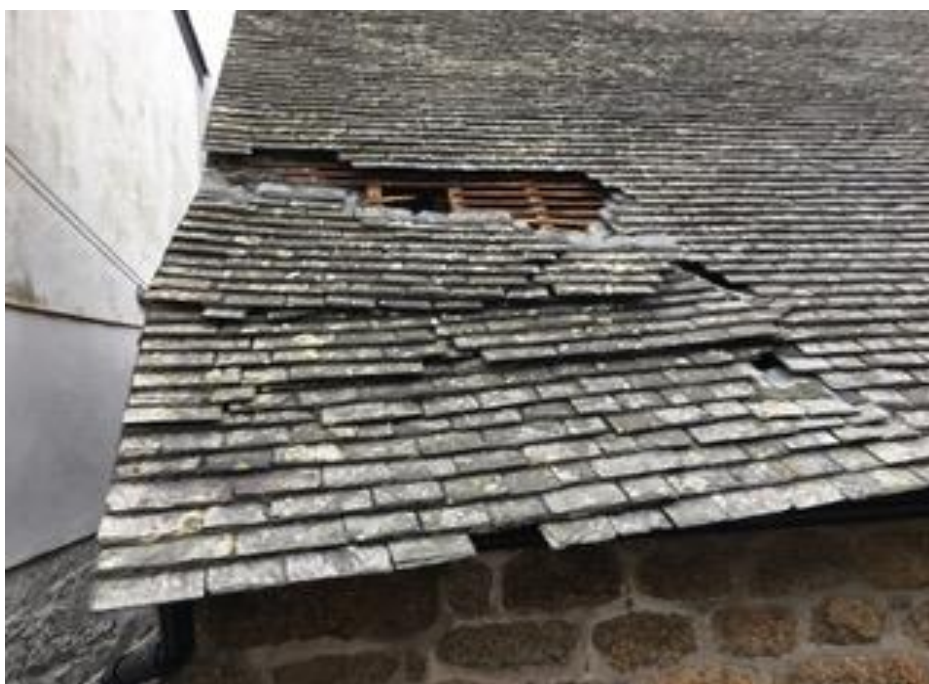
Fig. 4: Slippage of slates on the south roof of the rear south wing, in 2021 (Paul Osborne).
