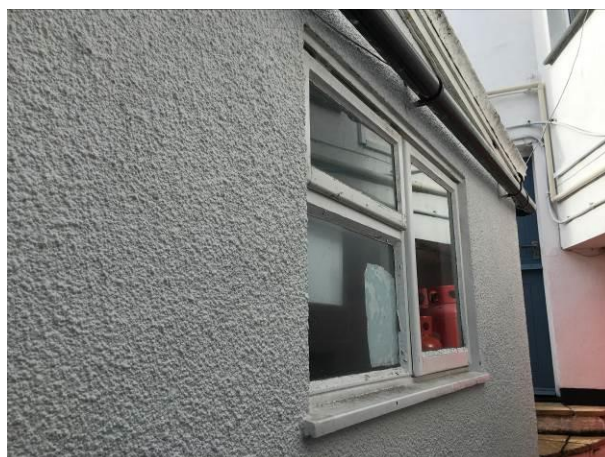
Photograph 8: Showing typical uPVC windows fitted tightly with rendering in good condition.
