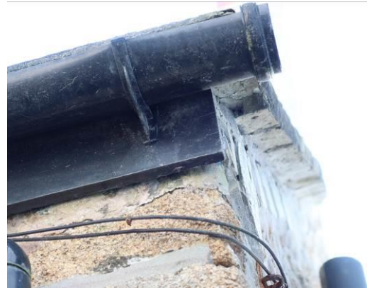
Photograph 2: Showing fascia board and guttering which runs along the eaves, along with the well-sealed gable end.
