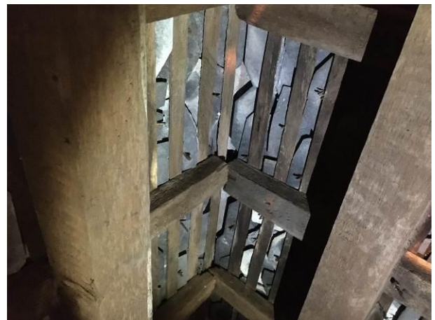
Photograph 6: Showing the internal pitch of the roof – no ridge board/beam is present.
