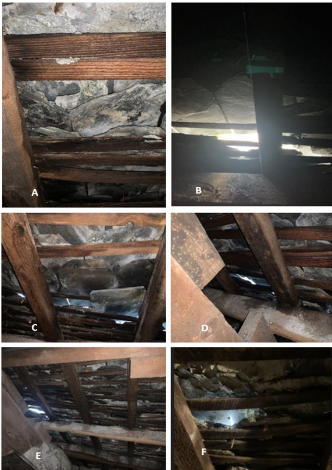
Fig. 15, A-F: Internal evidence of deterioration of roof battens and slate slippage.
