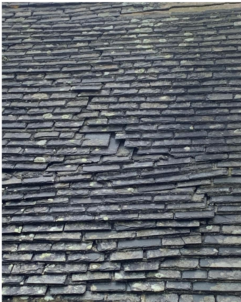
Fig. 16: Cumulative downward displacement of slates on the north-west side of the south wing of Kavorna.
