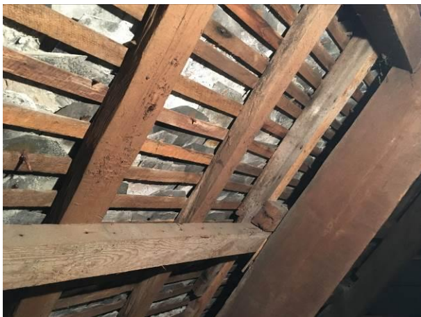
Photograph 5: Showing the interior of the loft space with scandle tiles laid directly onto timber battens – no underfelting present.
