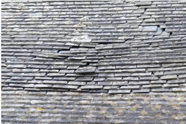
Photograph 3: Showing the areas of slipped tiles on the roof.
