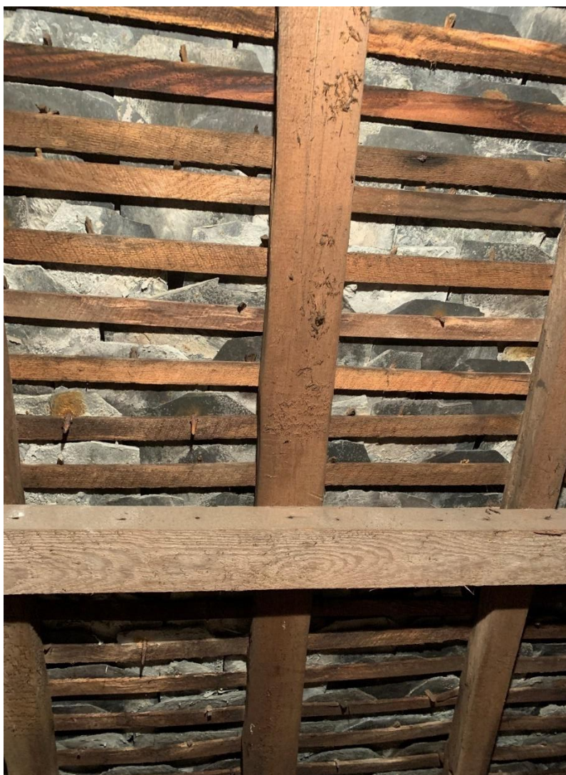
Fig. 14: Internal details of roof construction: purlin, common rafters and battens.
