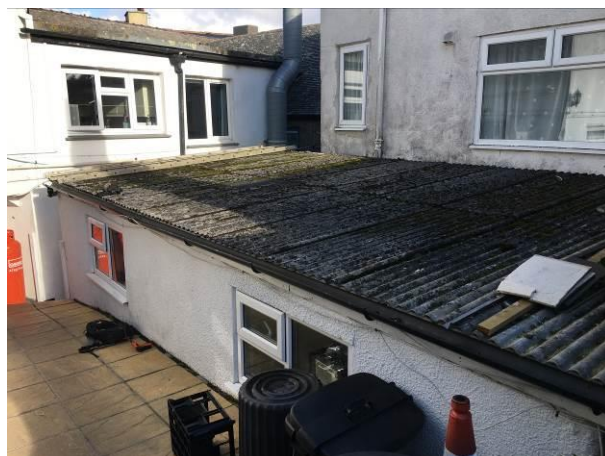
Photograph 10: Showing the western aspect with a pitched, corrugated roof.
