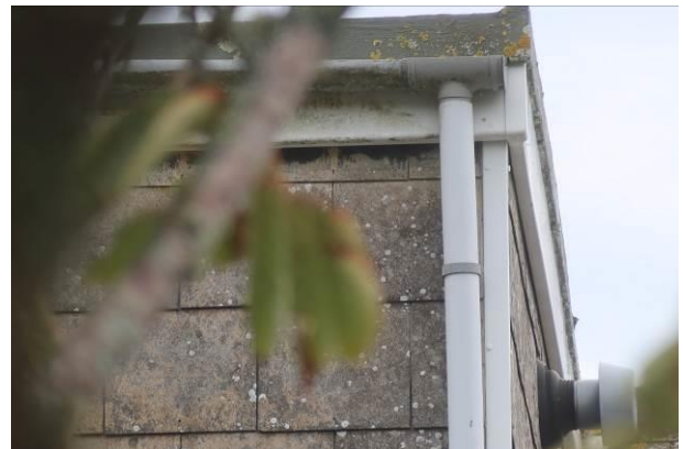
Photograph 6: Showing the well-fitted asbestos tiles on the front and side of the dormer window on the rear of the property.
