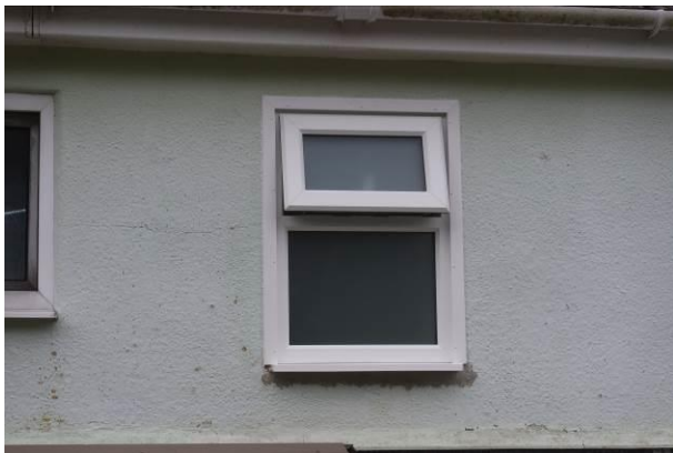
Photograph 5: Showing a typical example of a well-fitted uPVC window found throughout the property.
