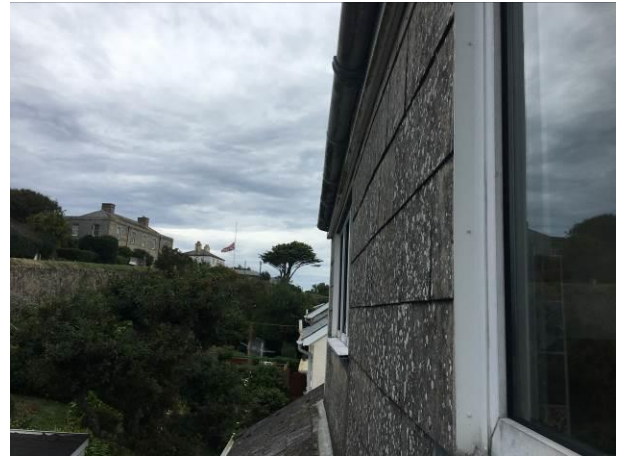
Photograph 8: Showing the hanging tiles on the dormer window viewed at height.
