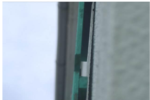
Photograph 4: Showing the battens attaching the shutters to the wall and the cavity created behind.
