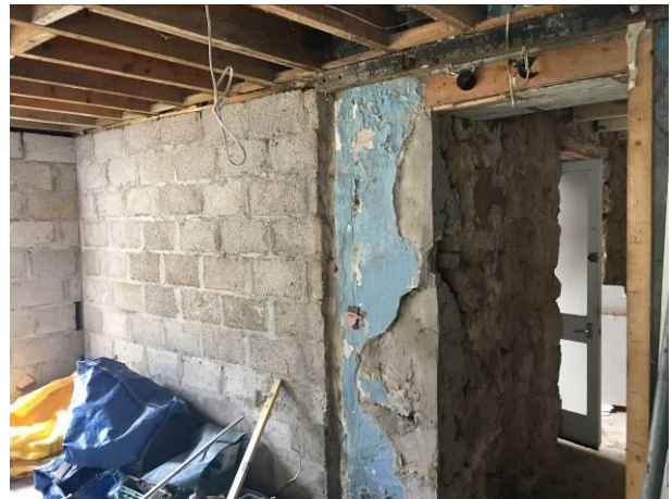
Photograph 10: Showing the interior of the garage with exposed breeze block walls and exposed timber roof structure above.
