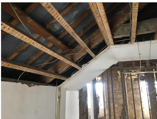
Photograph 5: Showing the interior of the roof of the main residential dwelling. This is the roof into which the new roof structure of the replacement bathroom dormer will be tied.
