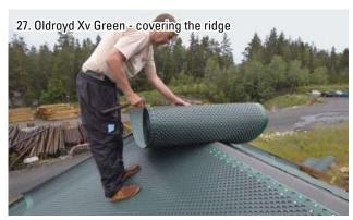
The final roll should be applied centrally over the ridge of the roof. Ensure overlaps are greater than the minimum requirement for pitch of roof (see step 23).
