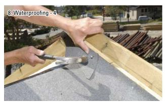
Apply a double layer of roofing felt over any joints, for example at the ends of the ridgeline.
