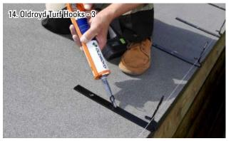
Seal around the fixing screws with Oldroyd sealing mastic.
