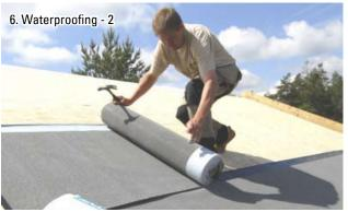
Working up the roof, roll out the next roll of roofing felt and tack into position. With temperatures less than around  $0^{\circ}$ C, warm the overlapping adhesive with warm air. It is inadvisable to use a naked flame.
