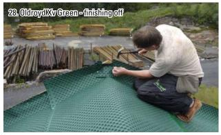
Cut small pieces of Oldroyd Xv Green membrane to cover any remaining odd-shaped areas, for example at the end of the ridgeline.
