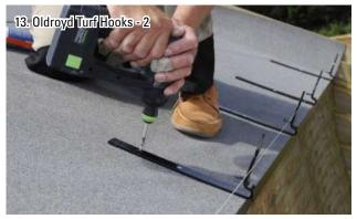
Turf hooks should be installed in line with the rafters, at spacings no greater than  $500\,\mathrm{mm}$ .
