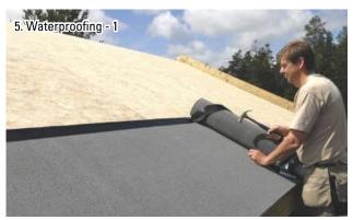
The roof should be waterproofed with a good proprietary bitumen-based roofing felt, for example Icopal Super D or similar BBA approved exterior grade. Roll out lengthways starting at the bottom (eaves) of the roof.
