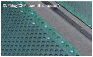
Fixings should be staggered with a minimum spacing of 400mm at pitches below 20°, and 200mm for over 20° pitch.
