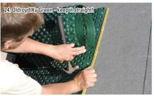
When working up the roof, ensure that the new layer remains parallel to the previous layer.
