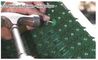
Secure the Oldroyd Xv Green membrane to the perimeter upstand with Oldroyd fixing plugs and nails.
