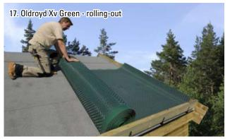
The Oldroyd Xv Green is rolled out over the roofing felt as shown.
