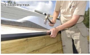
A neat and waterproof edge can be created by using an eaves drip tray. This is simply nailed into position under the waterproof roofing felt. Use Oldroyd sealing mastic to ensure that nail holes are sealed.
