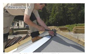
Ensure the roofing felt overlaps at the apex (ridge).
