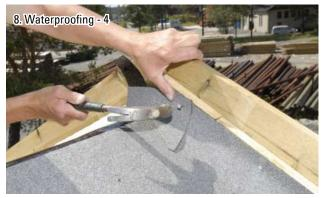
Apply a double layer of roofing felt over any joints, for example at the ends of the ridgeline.
