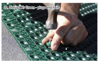
Oldroyd Xv Green is secured in position using nails and special Oldroyd turf roof plugs. The nails make a tight fit through the plugs which are designed to fit exactly within the membrane stud.
