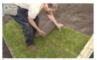
Finally the plants are installed. In this case, turf is being used and it is rolled out lengthways along the roof.
