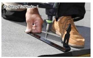
Front edging boards hold the growing medium in place and prevent it from slipping. The edging boards are secured to the roof using special Oldroyd Turf Hooks to ensure drainage is not impeded.
