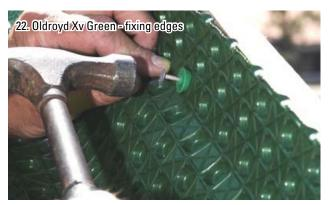
Secure the Oldroyd Xv Green membrane to the perimeter upstand with Oldroyd fixing plugs and nails.
