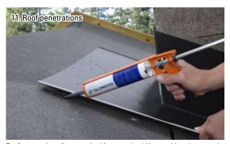
Roof penetrations, for example chimneys, should be considered separately. Use sections of the felt cut to size to form a neat seal. Chimneys can be sealed with the Oldroyd chimney collar. Again, use Oldroyd sealing mastic to complete the watertight seal.
