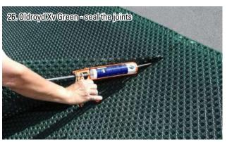
Apply Oldroyd sealing mastic at the edge of all horizontal and vertical overlaps to ensure a waterproof seal. Also use to seal all visible turf roof plugs and nails.
