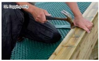
To stop water getting underneath the Oldroyd Xv Green membrane around the edge of the roof, a capping strip must be installed along the perimeter upstand.
