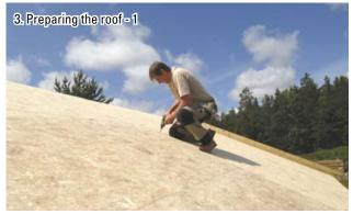
The roof would typically be constructed from timber, with the top surface boarded. Ensure roof and structure are strong enough to take the saturated weight of soil and plants (check with supplier).
