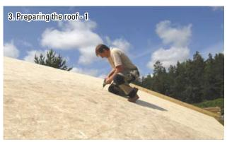
The roof would typically be constructed from timber, with the top surface boarded. Ensure roof and structure are strong enough to take the saturated weight of soil and plants (check with supplier).
