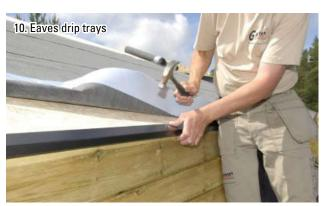
A neat and waterproof edge can be created by using an eaves drip tray. This is simply nailed into position under the waterproof roofing felt. Use Oldroyd sealing mastic to ensure that nail holes are sealed.
