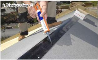
Use Oldroyd sealing mastic to seal thoroughly around visible tacks and any joints.
