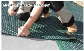
Continue up the roof, rolling out the next layer. There should be a minimum horizontal overlap of 300mm for under  $20^{\circ}$  pitch, and a minimum of 200mm for over  $20^{\circ}$  pitch.
