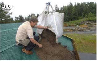
The roof soil is placed. A 300mm gravel border is recommended to provide ballast, prevent soil erosion at edges and act as a fire break.
