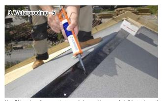
Use Oldroyd sealing mastic to seal thoroughly around visible tacks and any joints.
