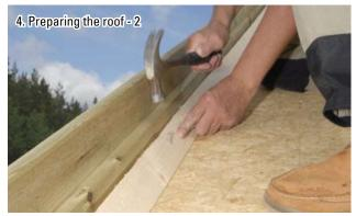
Champhered timber should be fixed along the perimeter upstands to ensure the roofing felt and membrane deflect water away from the edges.
