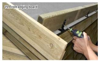
The front edging board is fixed to the turf hooks using screws.
