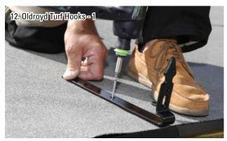
Front edging boards hold the growing medium in place and prevent it from slipping. The edging boards are secured to the roof using special Oldroyd Turf Hooks to ensure drainage is not impeded.
