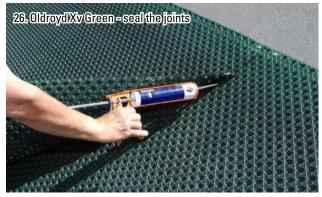
Apply Oldroyd sealing mastic at the edge of all horizontal and vertical overlaps to ensure a waterproof seal. Also use to seal all visible turf roof plugs and nails.
