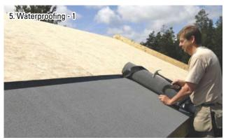
The roof should be waterproofed with a good proprietary bitumen-based roofing felt, for example Icopal Super D or similar BBA approved exterior grade. Roll out lengthways starting at the bottom (eaves) of the roof.
