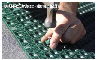
Oldroyd Xv Green is secured in position using nails and special Oldroyd turf roof plugs. The nails make a tight fit through the plugs which are designed to fit exactly within the membrane stud.
