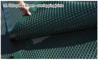
Ensure that all joints overlap. Vertical overlap should be at least 500mm.
