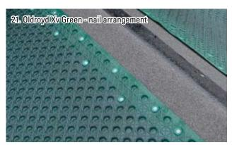
Fixings should be staggered with a minimum spacing of 400mm at pitches below 20°, and 200mm for over 20° pitch.
