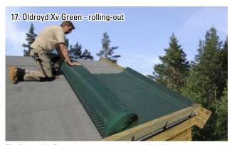
The Oldroyd Xv Green is rolled out over the roofing felt as shown.
