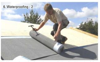
Working up the roof, roll out the next roll of roofing felt and tack into position. With temperatures less than around  $0^{\circ}$ C, warm the overlapping adhesive with warm air. It is inadvisable to use a naked flame.
