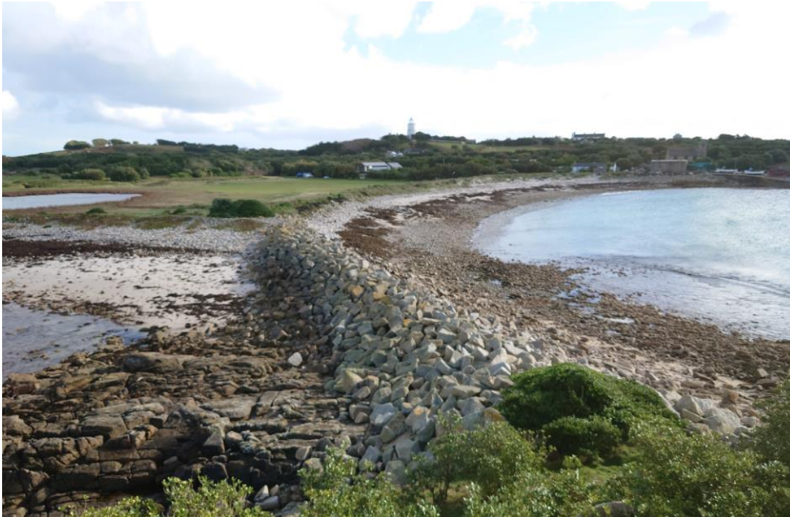
Figure 1-17: Formal rail and boulder groyne from Ginamoney Carn to the point between Porth Coose and Periglis beach
