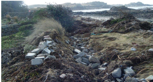
Figure 4-24: Over washed garden wall at Stinking Porth in 2014 (Ambios Environmental Consultants Ltd 2014)
