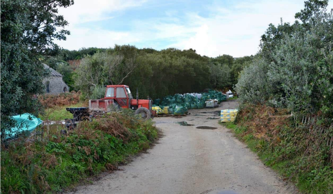
Photograph 6 (Bryher): building materials compounds
