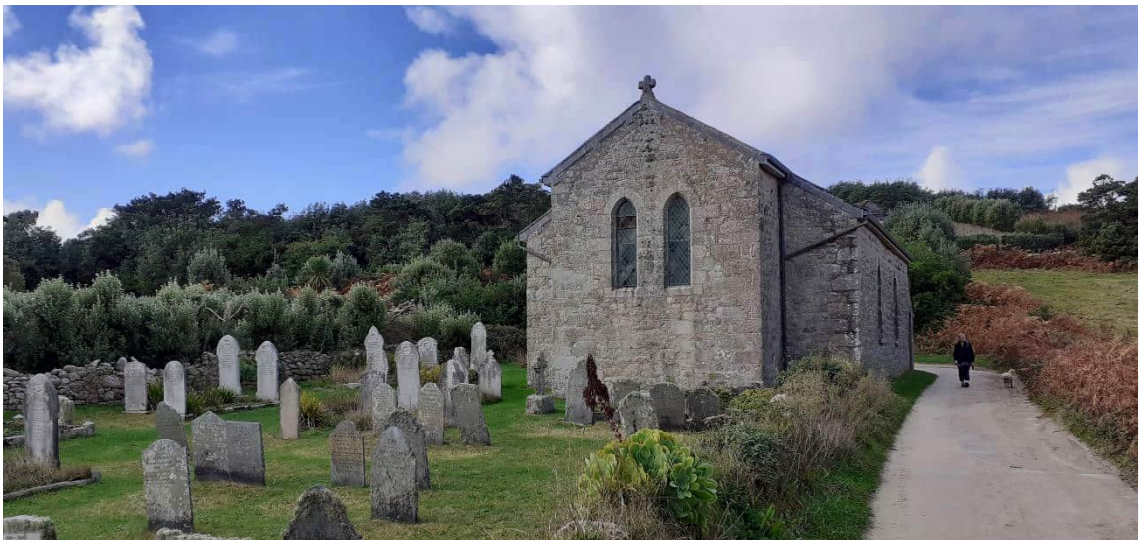
Photograph 12: Grade II listed Church of All Saints (1141234)
