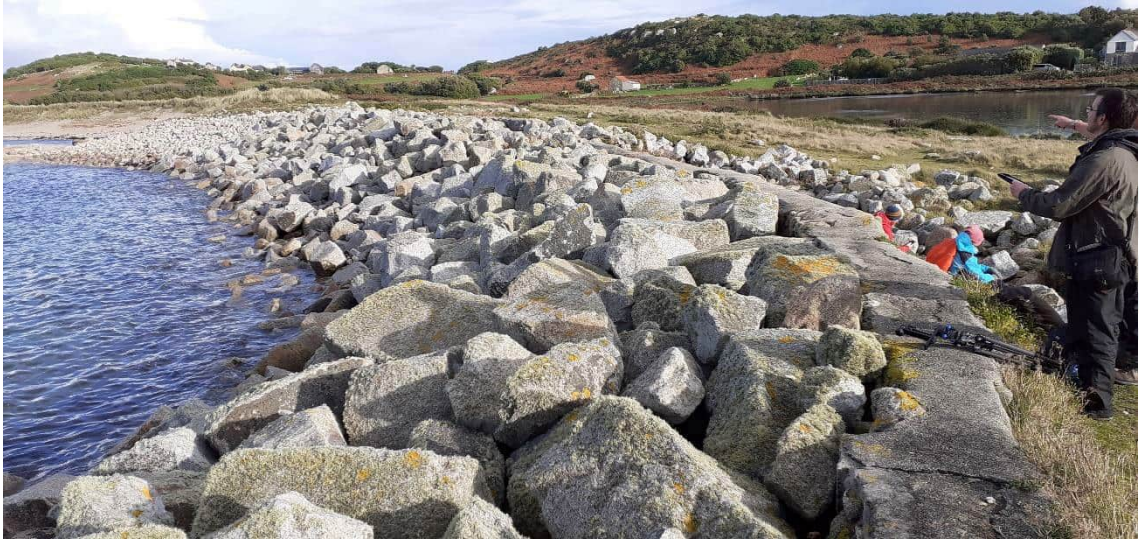
Photograph 9: View looking east across Popplestones site showing current rock armour and concrete sea wall
