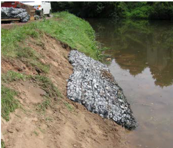
Pre-filled Rock Mattress installation before and after
