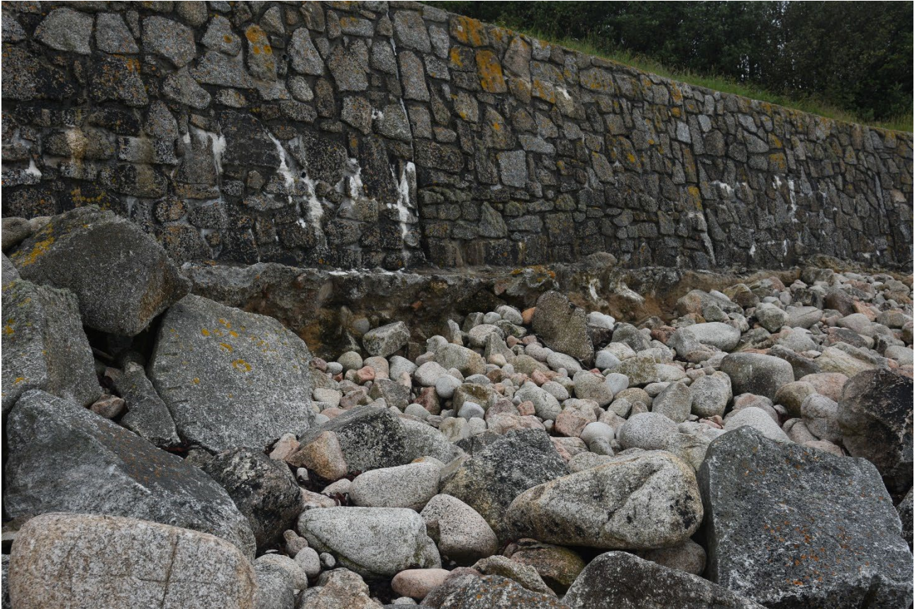
Photograph 5.1: Porth Killier exposed sea wall footing
