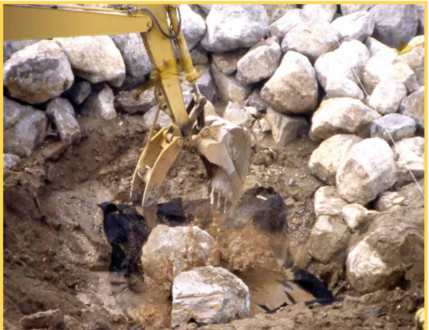
▲ Live Installation: 3t rock armour dropped from 2m height onto HPS14 overlying a sandy clay unconsolidated beach deposit.
