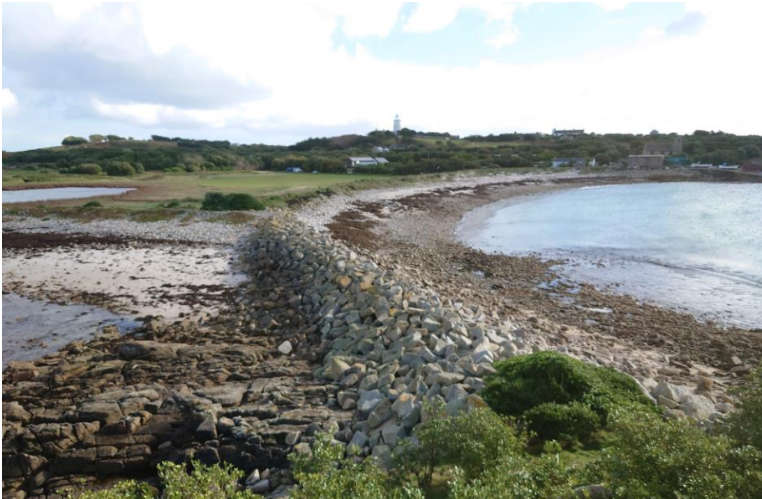
Figure 15: Former rail and boulder groyne from Ginamoney Carn to the point between Porth Coose and Periglis Beach.
