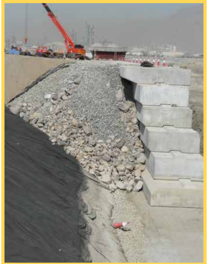
Case Study: Hulayla Marina Development. HPS filter/seperator geotextiles preventing intermixing of fill layers behind quay wall structure.
