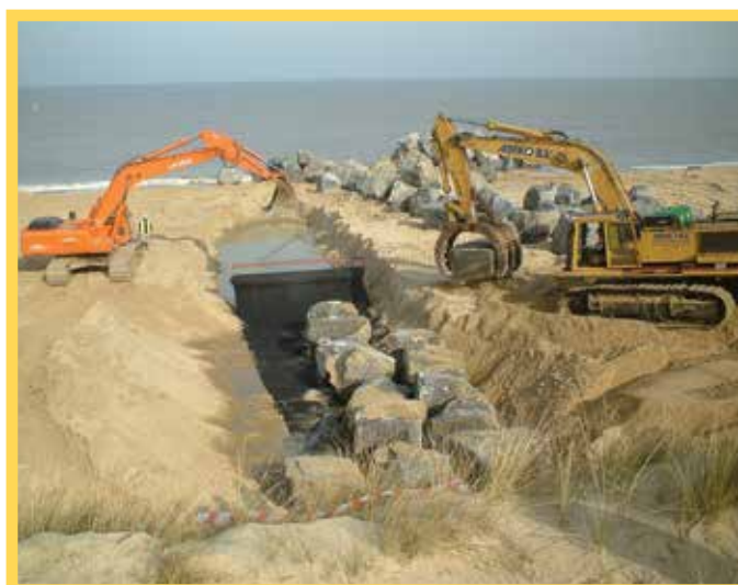
Rock armour Groyne installation to inhibit 'Long Shore Drift' and protect the coastline.
