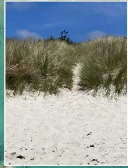
G SITE 27, Example of dune access erosion
