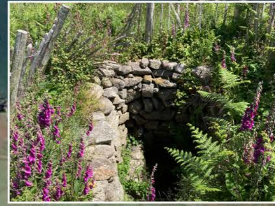
E SITE 27. Water intake location
