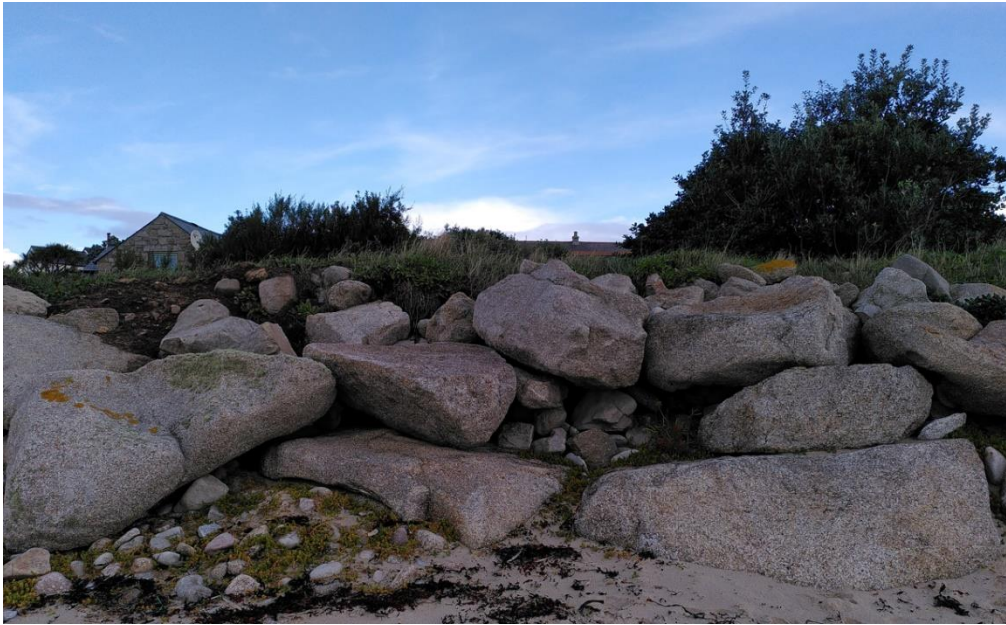
Figure 1-10: Protection provided by 1-3 tonne stones along the frontage of Great Porth
