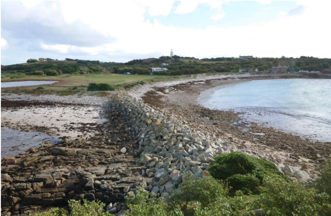
Figure 1-17: Formal rail and boulder groyne from Ginamoney Carn to the point between Porth Coose and Periglis beach
