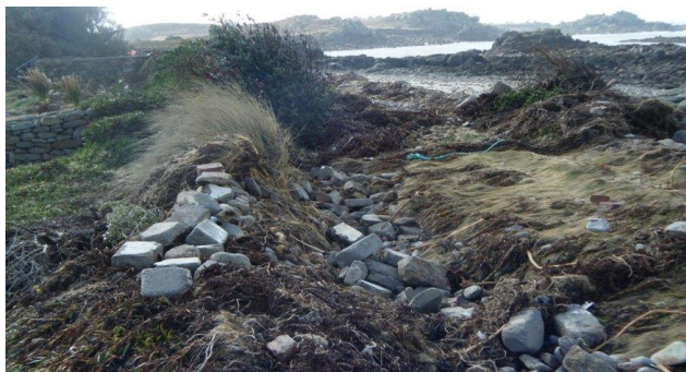
Figure 4-24: Over washed garden wall at Stinking Porth in 2014 (Ambios Environmental Consultants Ltd 2014)
