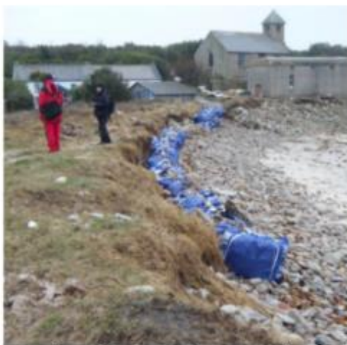
Figure 4-32: Sand filled bags placed around eroded dunes (JLA 2014)
