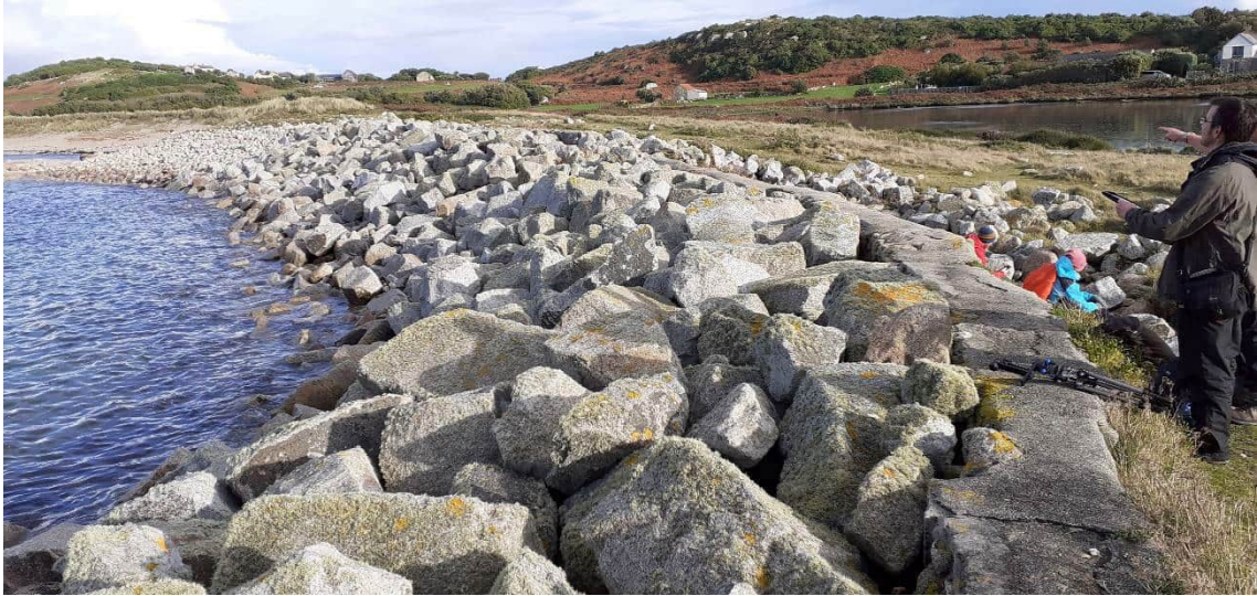
Photograph 9: View looking east across Popplestones site showing current rock armour and concrete sea wall
