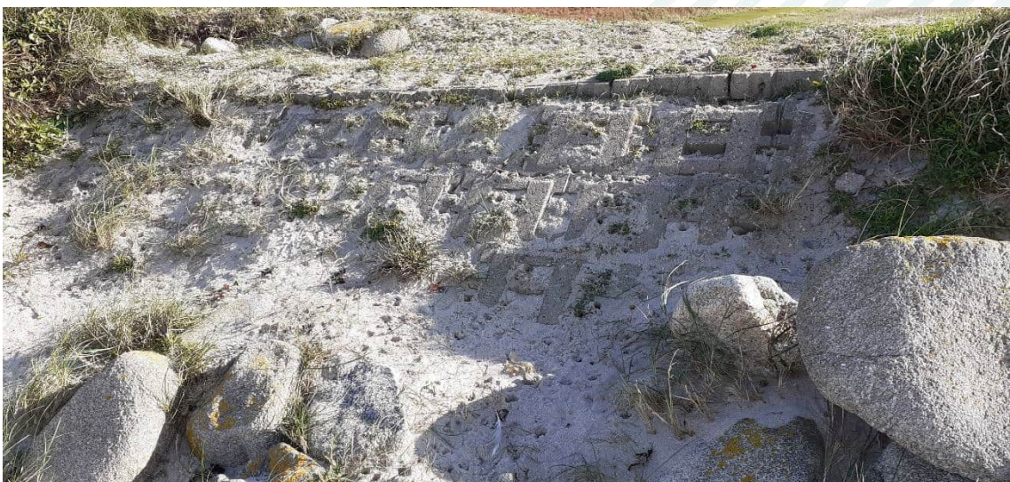
Photograph 21: Area of exposed concrete sea wall (MCO64519)
