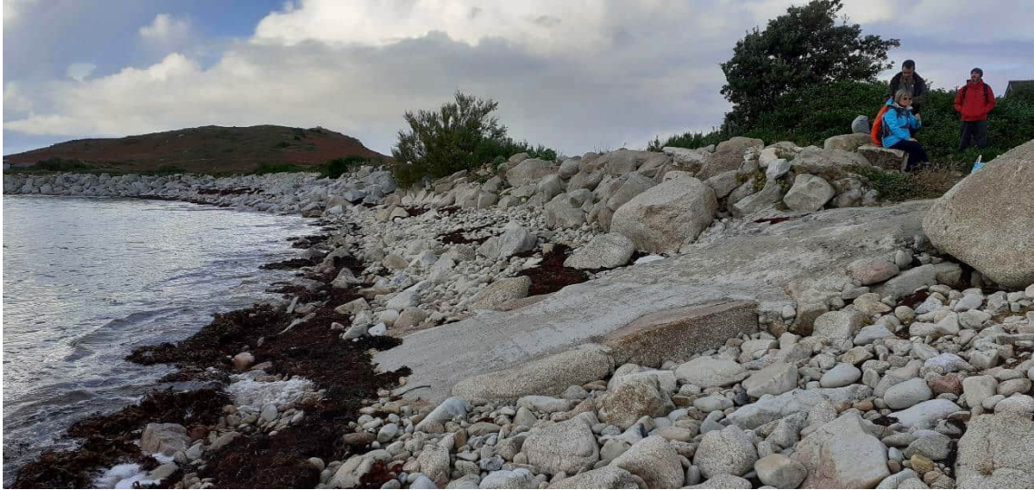
Photograph 6: View looking north west at Great Par site. Concrete slipway can be seen in the foreground.
