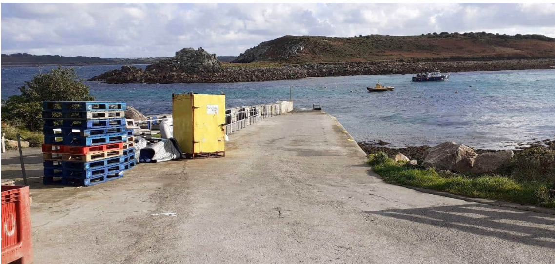
Photograph 14: Quay on St Agnes
