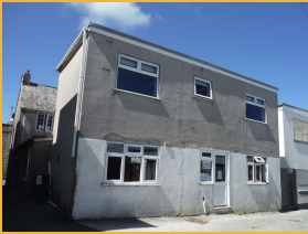
Photograph of the rear of the building – assumed extension from the early 1980's. Considered to be of poor architectural quality.
