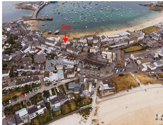
Aerial Photograph of Steamship House From South East
