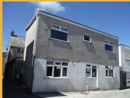
Photograph of the rear of the building – assumed extension from the early 1980's. Considered to be of poor architectural quality.
