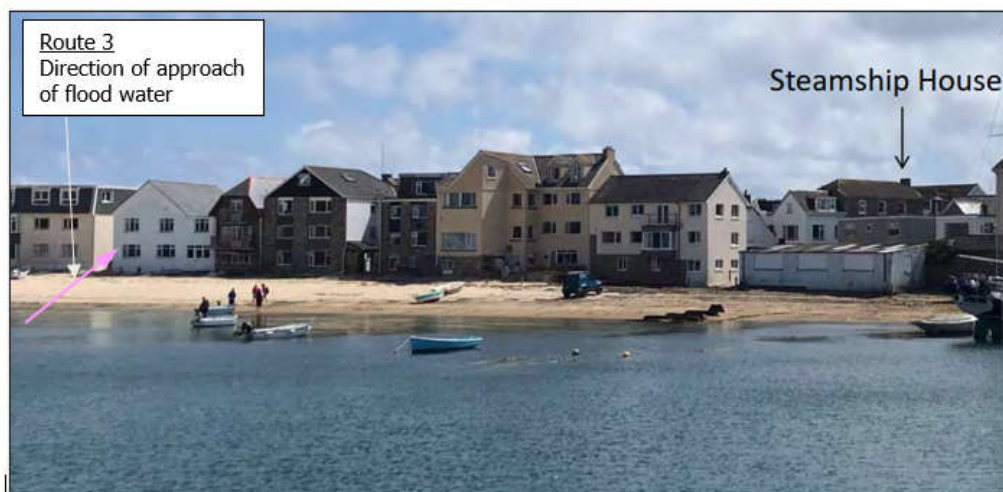
Photo 3 View Showing Potential Flood Routes to Side of Golden Bay Mansions
