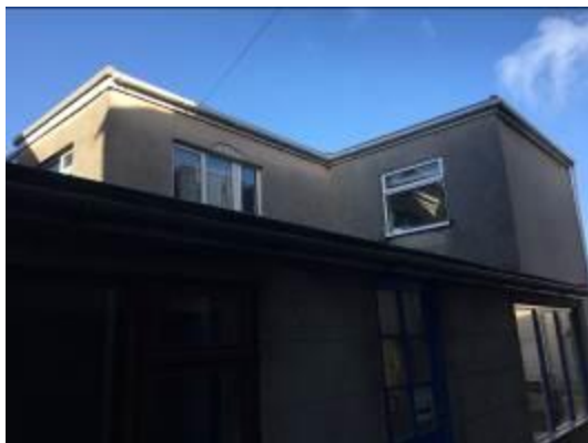
Photo 02 – Showing the pitched-roof single-storey building (B) in the foreground, with the two-storey, flat-roofed building (C) in the background.
