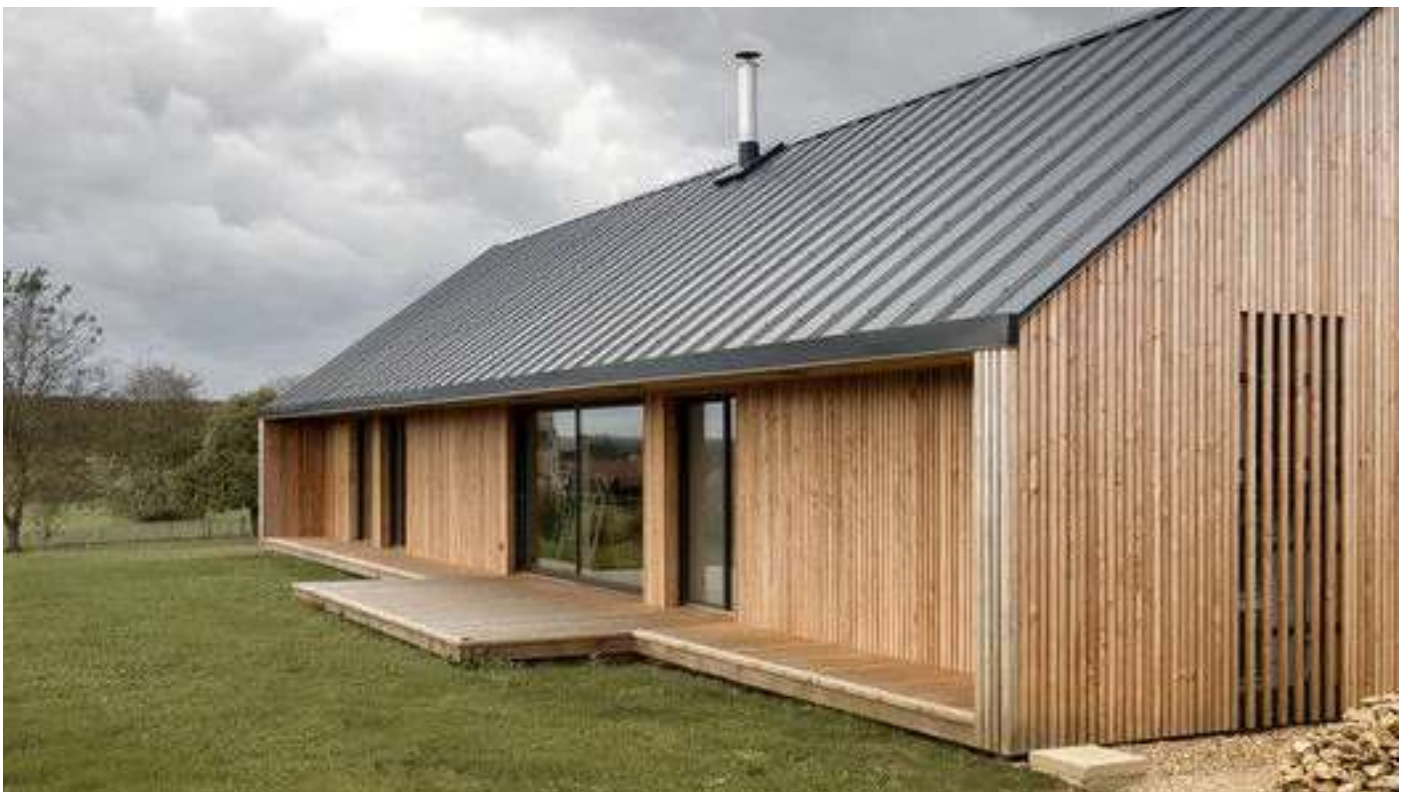
A simple palette of materials, including timber cladding, standing seam metal roofing and timber decking
