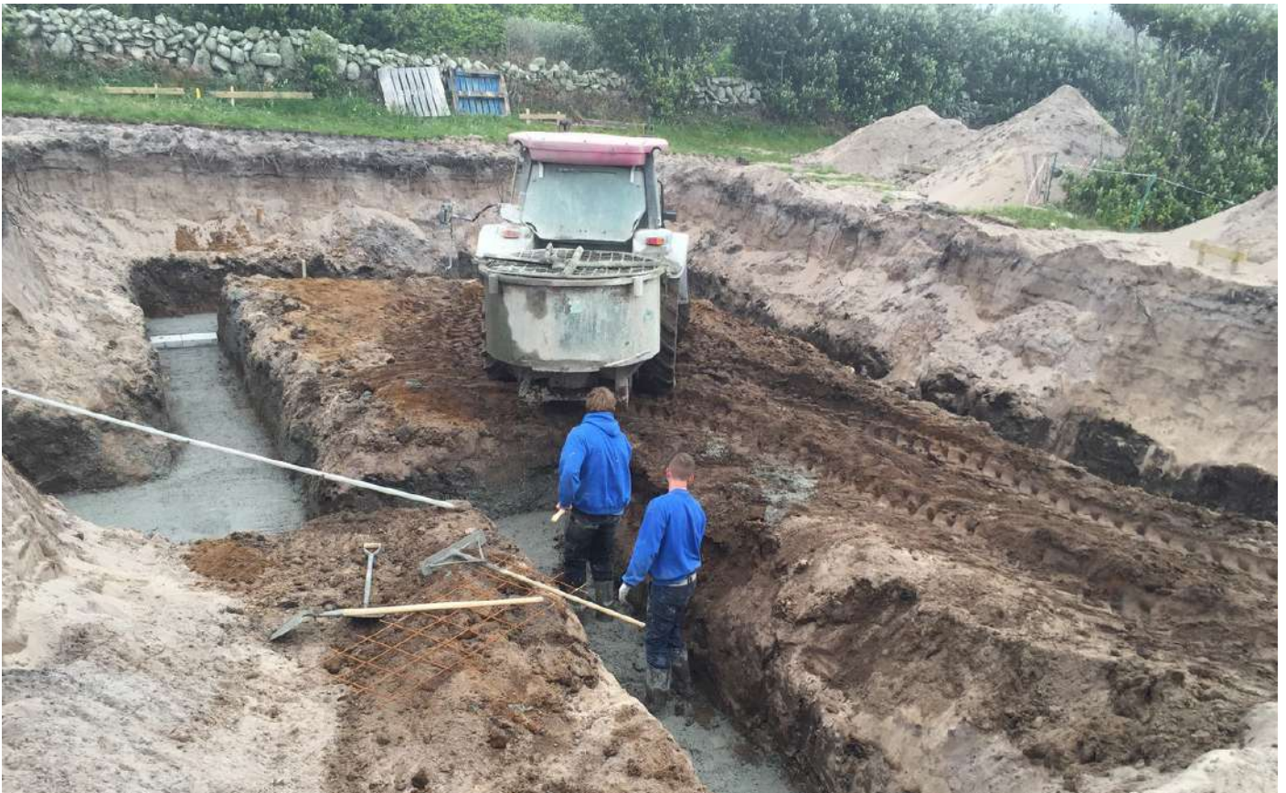
Digging for foundation of the new build at Trethagan, adjacent to proposed site, showing the soil profile of the area. Top layer is approx 6 ft of wind blown sand. This is approx. 35m from the proposed location of the proposed shop.
