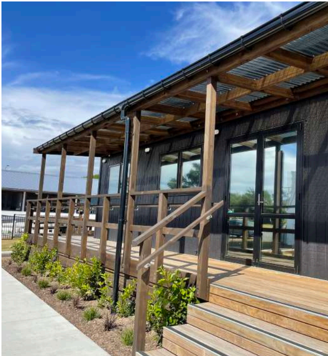
A Southern roof overhang to provide solar shading and protection from the weather
