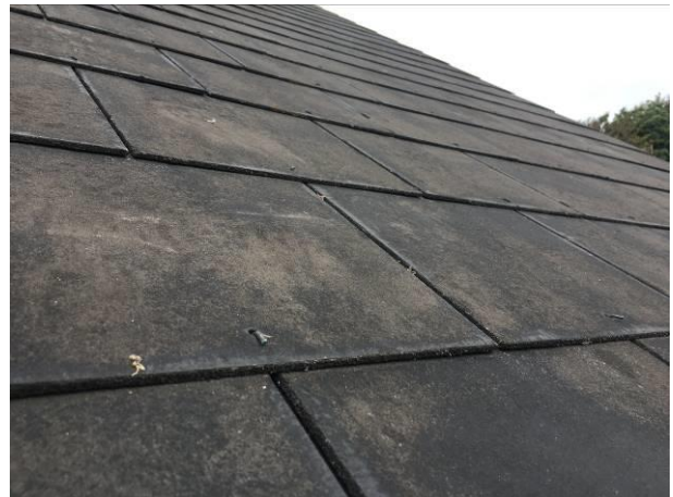
Photograph 4: Showing the tightly fitted slate roof on the existing property. This is the retained roof into which the new roof structure of the bathroom dormer will be tied.
