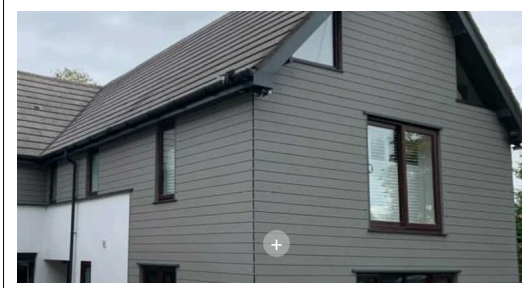
Cladco Stone Grey composite cladding to match house
