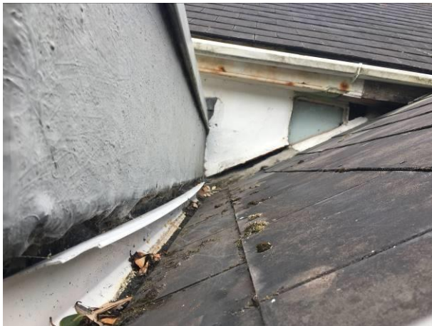
Photograph 3: Showing the existing gully between the fibre-glassed back wall of the dormer and the slate roof of the main property
