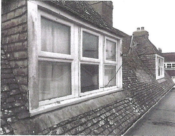
Photograph 1: Showing the pitch of the roof as viewed from the adjacent flat roof.
