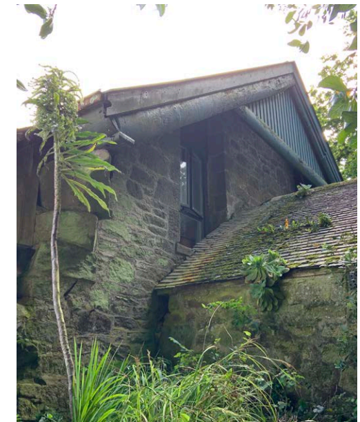
Figure 14. Scantle Roof Detail
