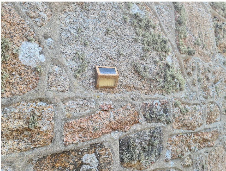
Figure 9: fitting marked for removal.
