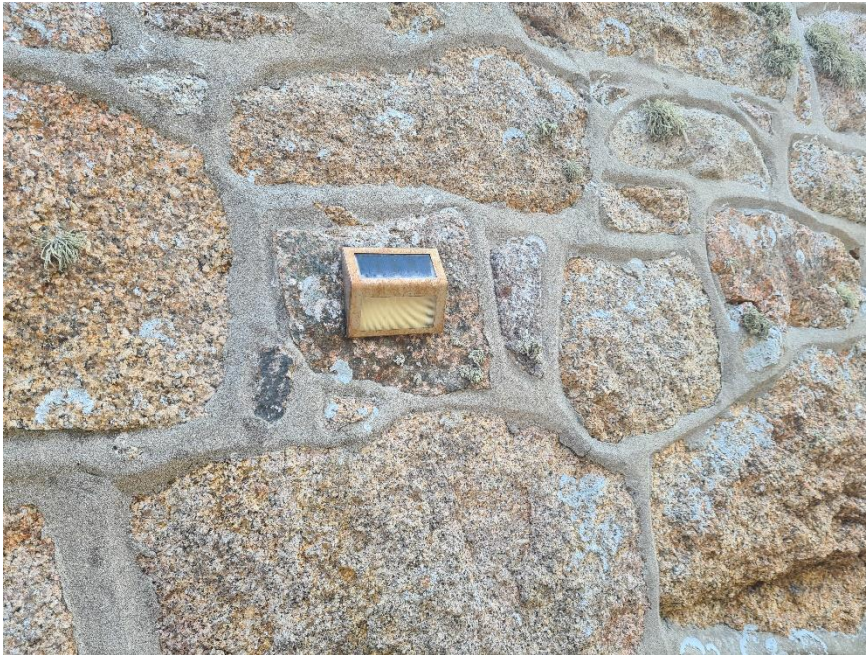
Figure 8: fitting marked for removal.
