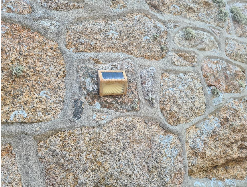
Figure 8: fitting marked for removal.
