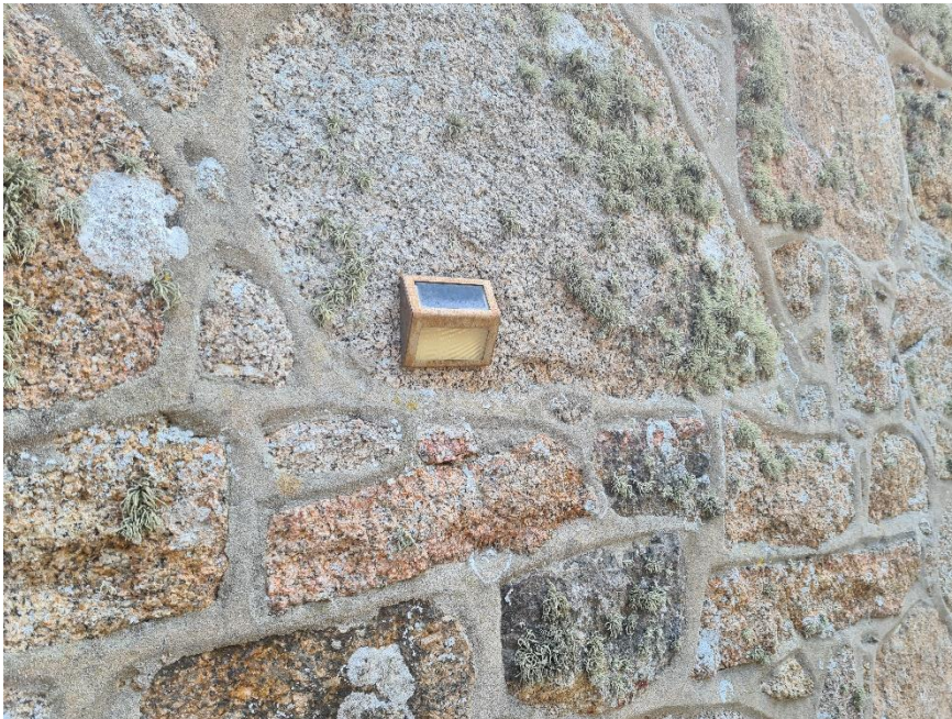
Figure 9: fitting marked for removal.
