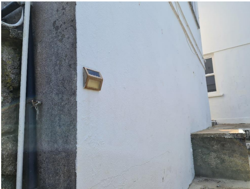
Figure 13: fitting marked for removal.
