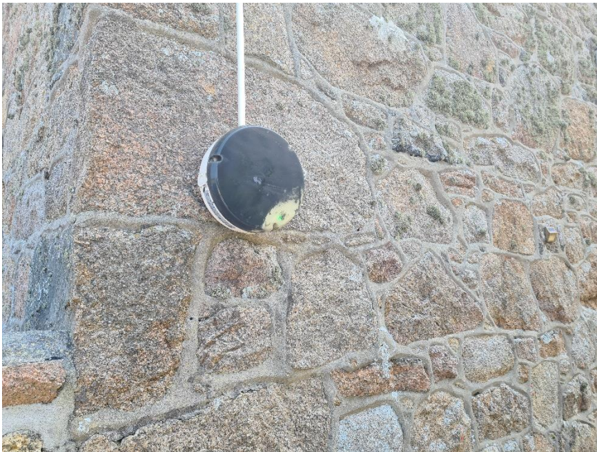
Figure 6: fitting marked for removal.
