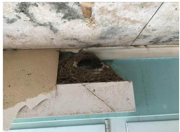
Photograph 6: Showing an example of one of the birds nests within the property, resulting from lack of occupation.
