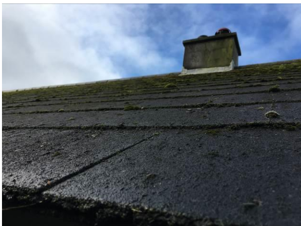
Photograph 5: Showing the tight fit of the roof tiles, with no gaps noted throughout.
