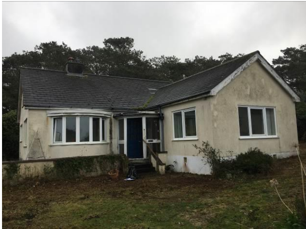
Photograph 1: Showing the main existing dwelling on the site.
