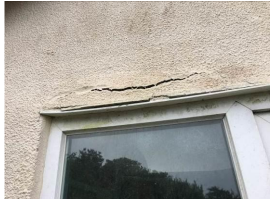
Photograph 6: Showing an example of the well-fitted window frames with no gaps or crevices. Cracks and damage in the render, as illustrated, are superficial and not suitable to support bats.
