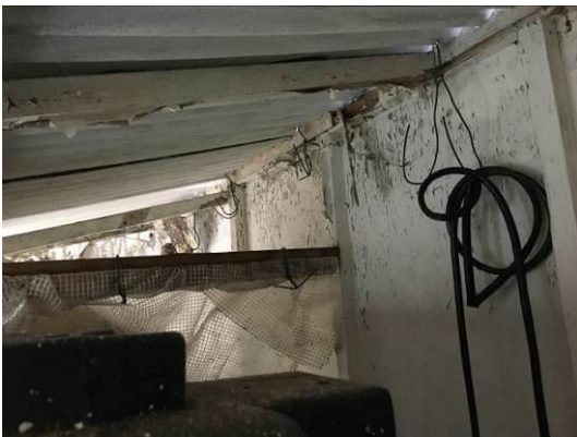
Photograph 15: Showing the roof of the canopy sheltering the oil tank.
