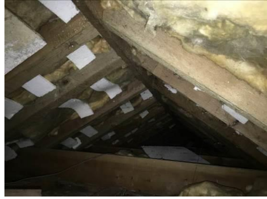
Photograph 12: Showing the main loft above the tie-beam in the main dwelling.
