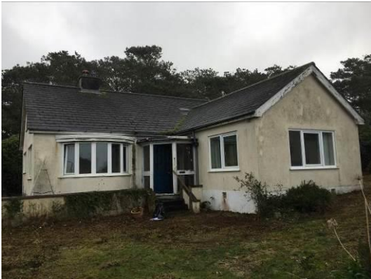
Photograph 5: Showing the main existing dwelling on the site.
