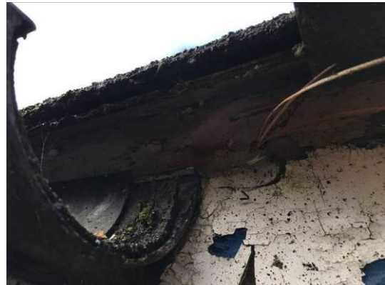
Photograph 8: Showing an example of the eaves where the guttering is displaced, demonstrating the lack of access for bats.
