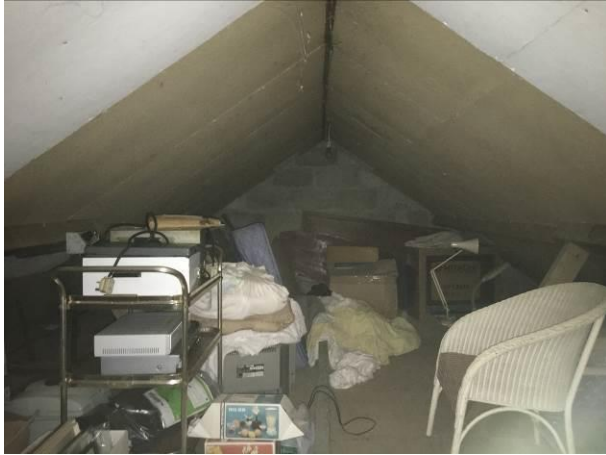
Photograph 7: Showing the interior of one of the boarded out loft components within the property – this example is at the apex but those at the eaves are of equivalent construction.
