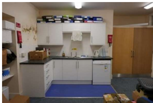
Ground floor kitchenette
