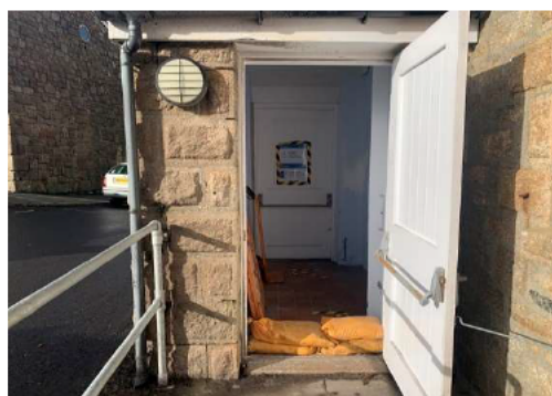
Rear entrance with sandbags across threshold.
