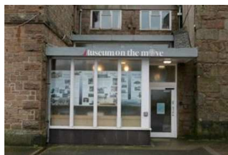
New public entrance off Church Street
