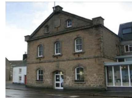
Front of Town Hall: view from Church Street
