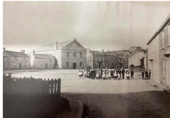
Figure 6: Undated photograph shortly after construction of the Town Hall © Isles of Scilly Museum Archive
