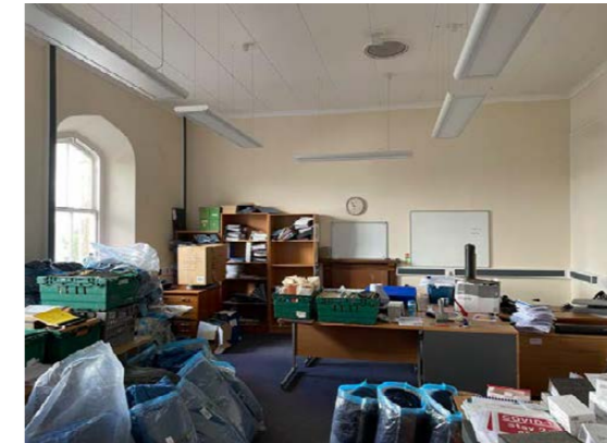
Figure 15: The former chamber/magistrates court with modern ceiling tiles, strip lighting and modern fire surround (2021)
