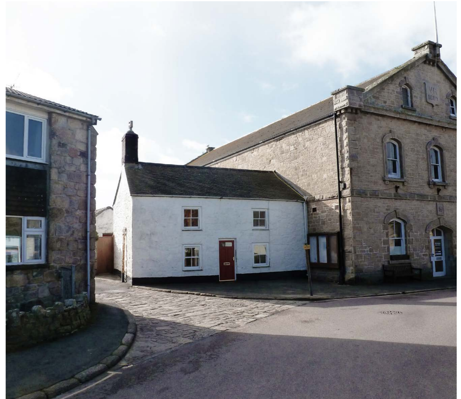
North east elevation of Parade Cottage
