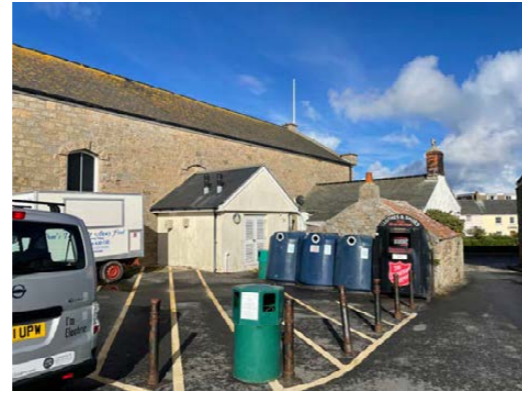
Figure 20: The rear of Parade Cottage and the Town Hall.
