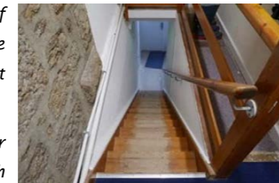
Emergency escape stairs leading to rear of building
