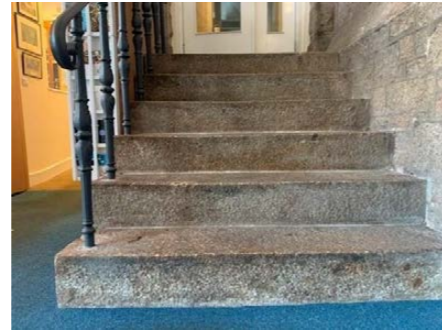
Stone staircase from main reception to other parts of the building
