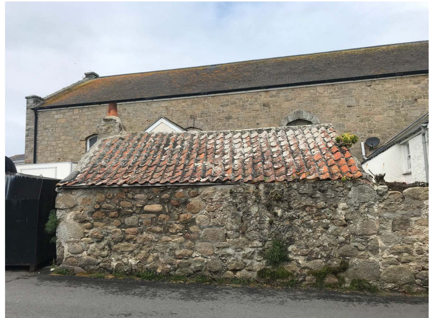
The south east elevation of the Outbuilding
