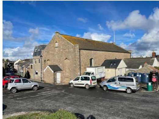
Figure 22: Rear of the Town Hall 2021
