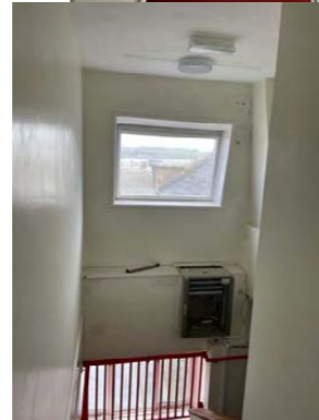
Figures 23&24: Internal space in the side extension
