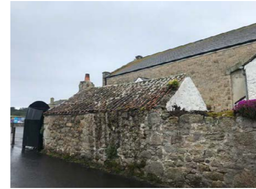
Rear small single storey structure (2023)
