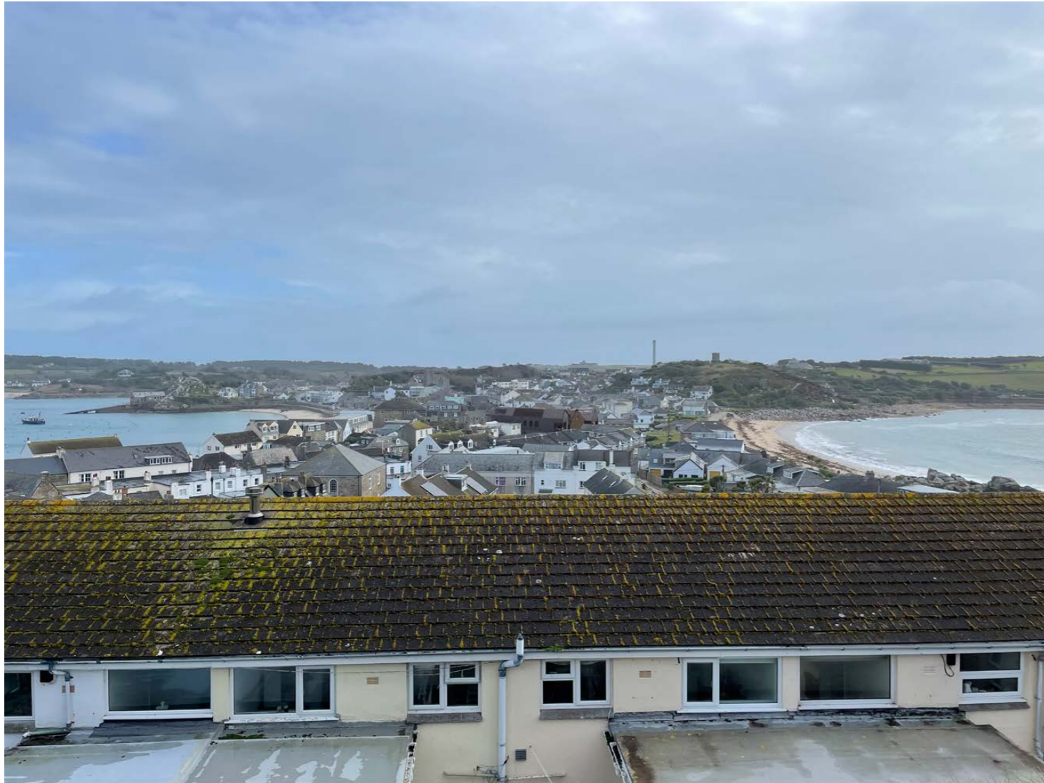
View from the Garrison over looking Hugh Town with the CGI image of the Town Hall added to the photo
