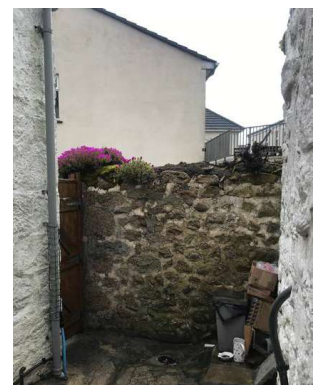
The external wall between Parade Cottage and the Outbuilding
