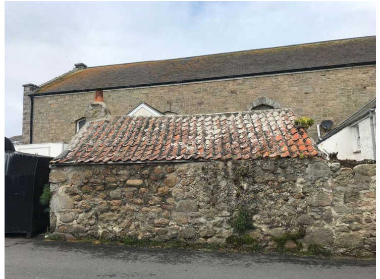
The south east elevation of the Outbuilding
