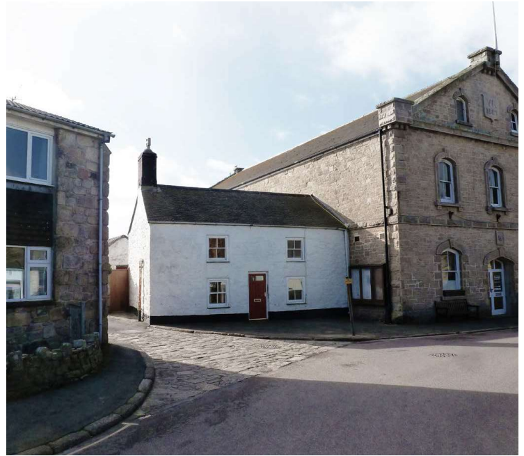
North east elevation of Parade Cottage
