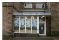
New public entrance off Church Street
