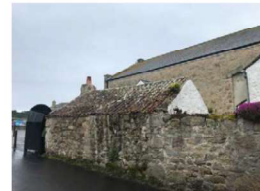
Rear small single-storey structure (2023)
