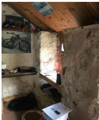
Inside of the Outbuilding
