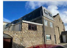
Figures 12&13: The 1970s extension on the western side of the Town Hall
