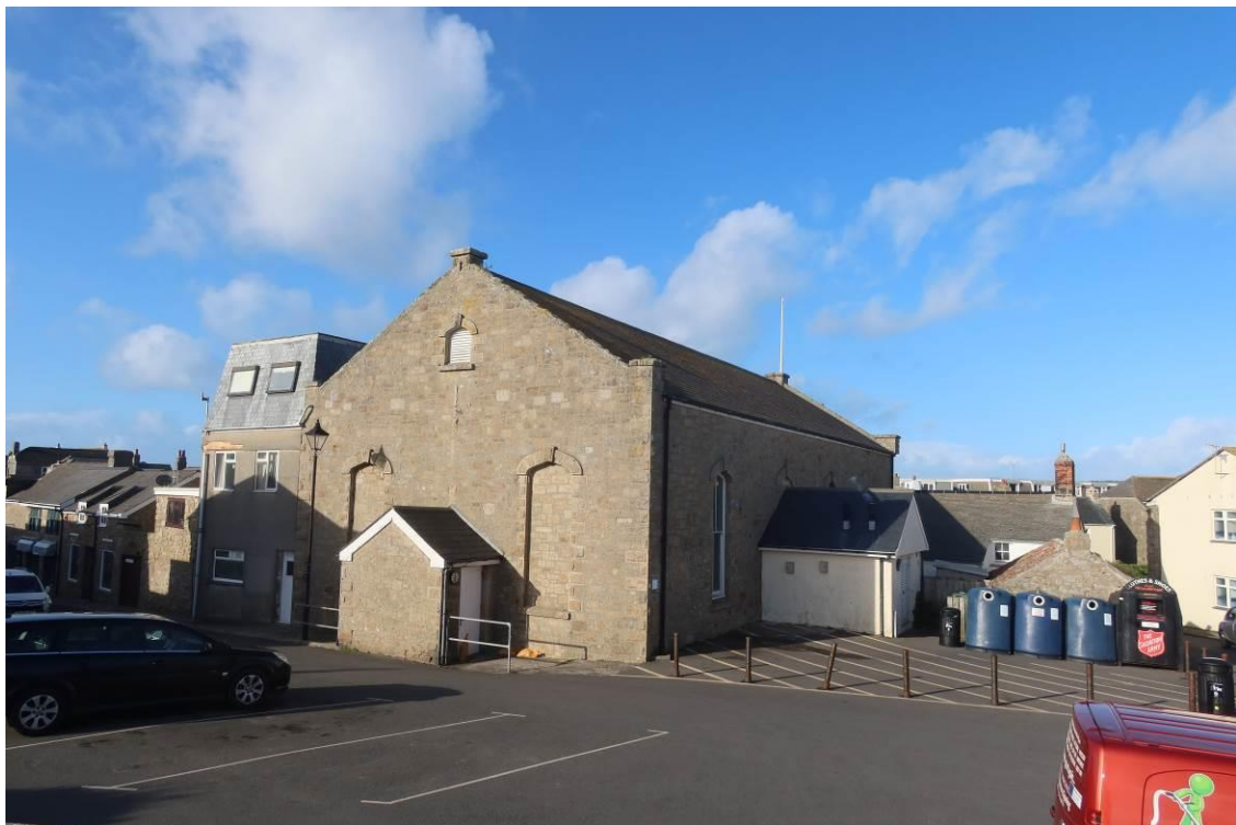
Photo 01 – Showing the main town hall building with the plant room to the right; the rear porch and the more modern extension to the left. The cottage and stone shed can be seen behind the glass collection point to the right of the photograph. The area of hardstanding included in the proposed development is the hatched area enclosed by bollards visible to the right.
