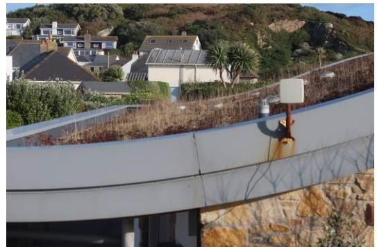
Photo 05 - Showing the sedum roof of the Tourist Information Centre.
