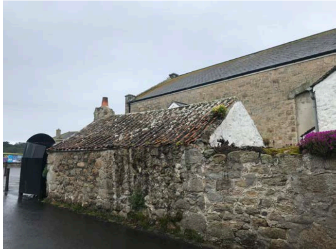
Rear small single storey structure (2023)
