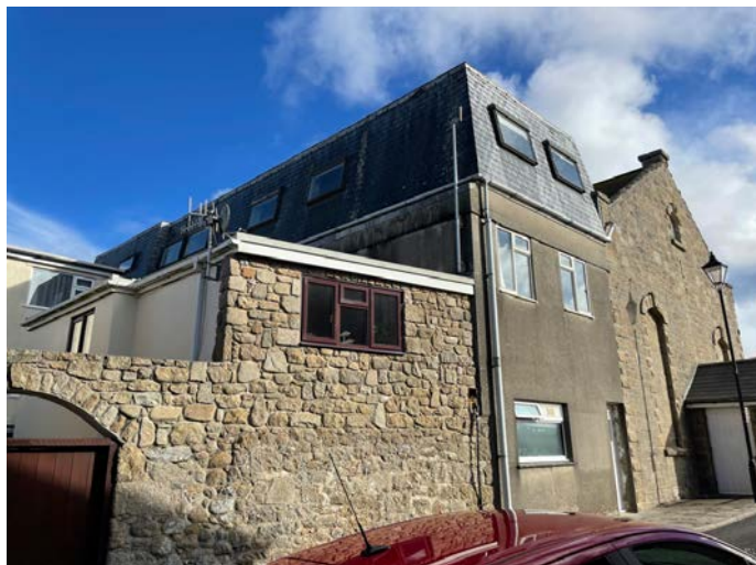
Figures 12&13: The 1970s extension on the western side of the Town Hall
