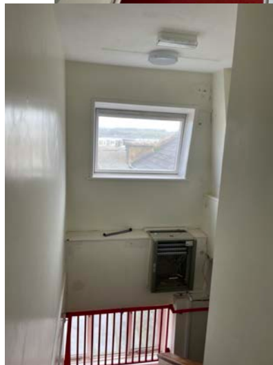
Figures 23&24: Internal space in the side extension
