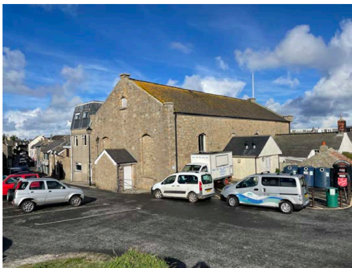
Figure 22: Rear of the Town Hall 2021
