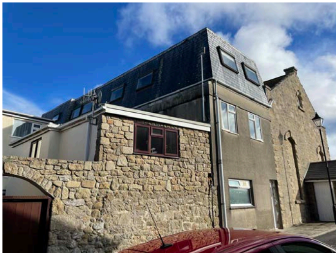
Figures 12&13: The 1970s extension on the western side of the Town Hall
