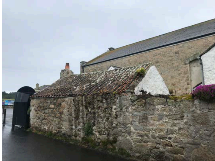
Rear small single storey structure (2023)
