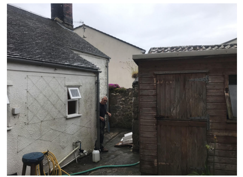
Photo of the yard showing the existing kitchen extension to Parade Cottage
