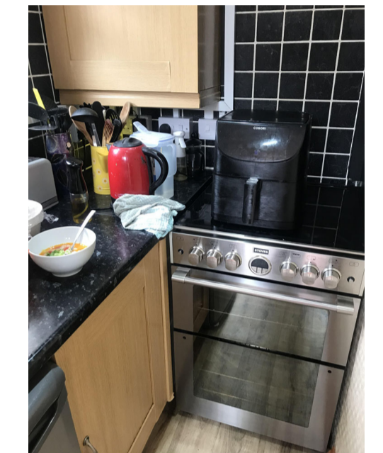
Cooker to be relocated to allow for new opening into the utility room
