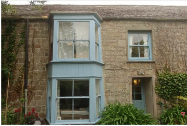
Photograph 1: Showing the front of the building with the bay windows visible.
