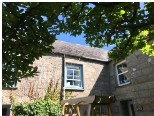
Photo 04 – Showing Magnolia Cottage from the exterior. The southern and western pitches of the roof can be seen.
