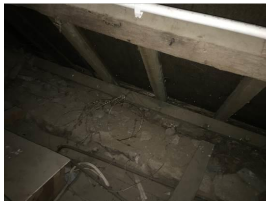
Photo 02 – Showing the eaves of the loft space
