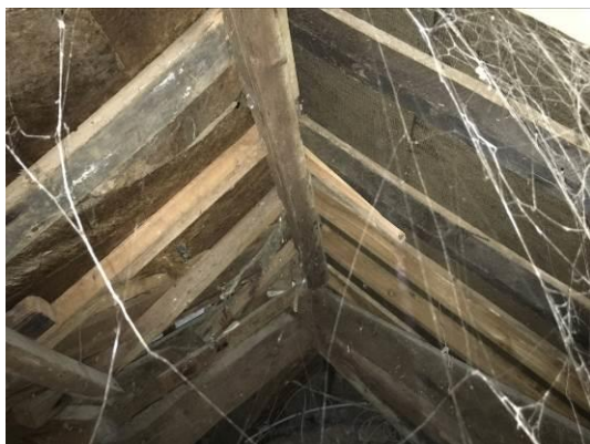
Photo 03 – Showing the timber roof structure with underfelting above
