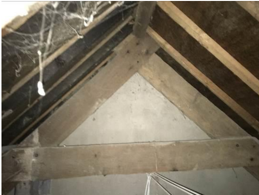
Photo 01 – Showing the terminal timber A-frame adjacent to the wall
