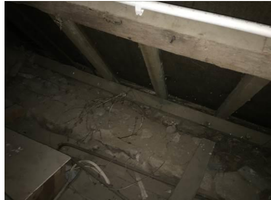
Photo 02 – Showing the eaves of the loft space
