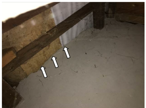
Photograph 6: Showing the concrete wall between Camelia and Magnolia Cottages with minor gaps at the top which a bat could potentially use to access between the loft spaces.
