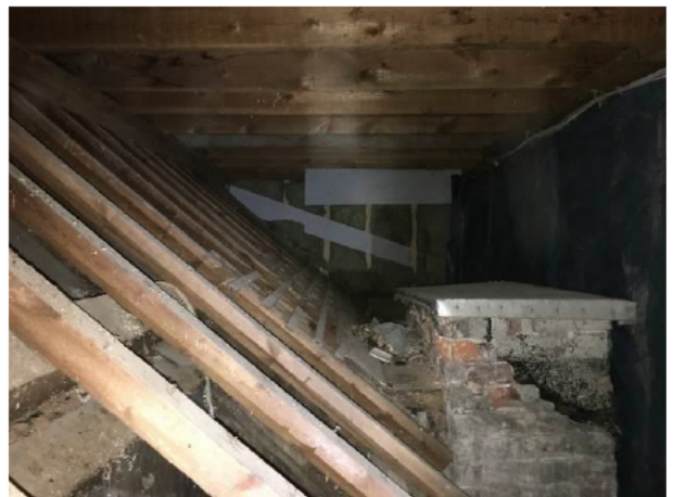
Photograph 4: Showing the redundant northern roof structure sealed within the flat-roof extension on the northern aspect of the building. Accessed and visible from the loft space of the property.
