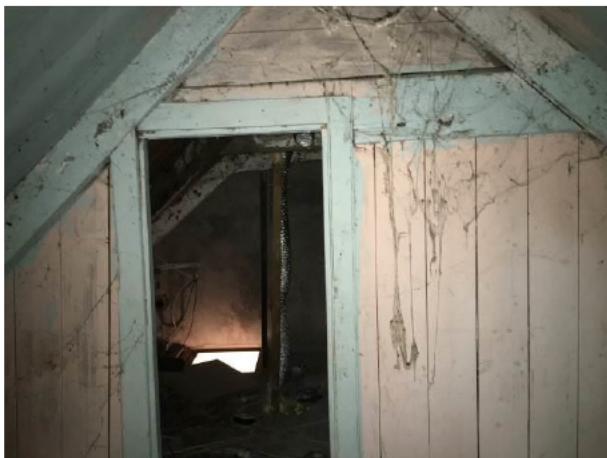
Photograph 3: Showing the timbers which underboard the loft space and also create an internal partition.
