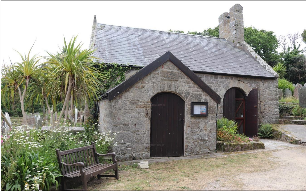
FIGURE 16: OLD TOWN CHURCH, FROM THE NORTH.
