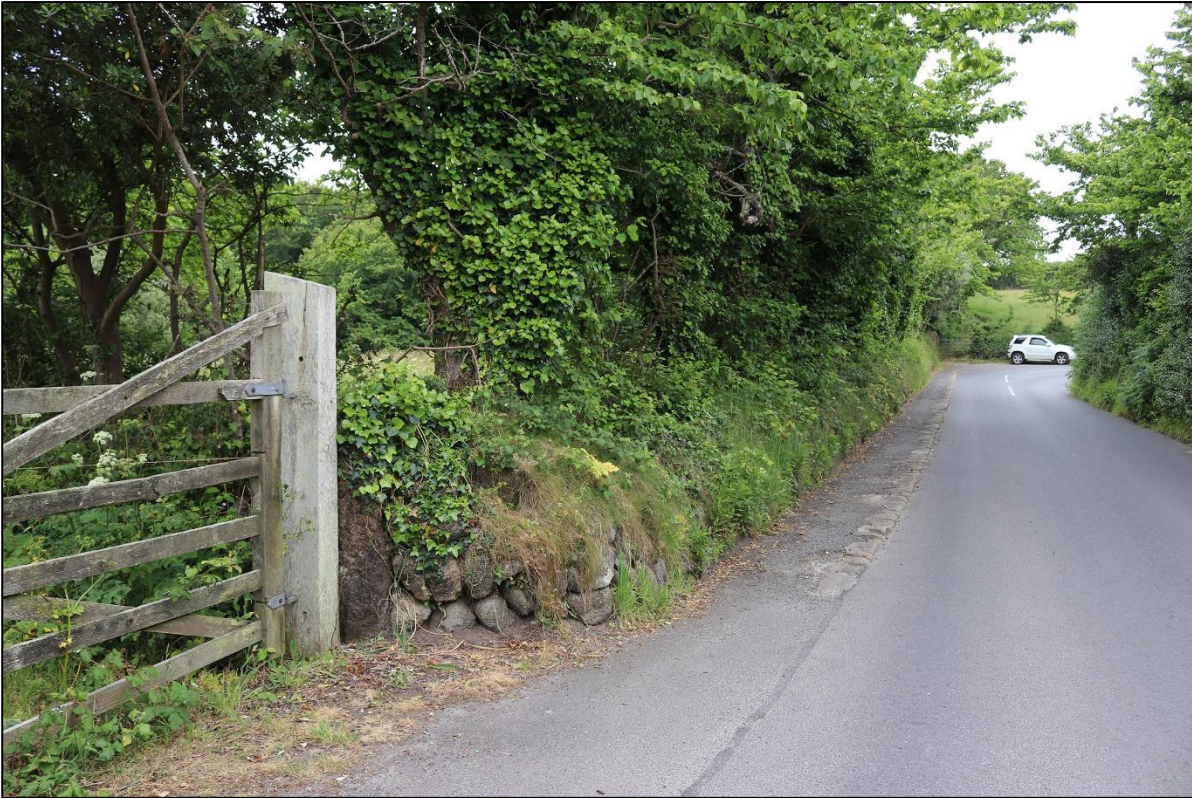
1. THE NORTH BOUNDARY LINING OLD TOWN ROAD; VIEWED FROM THE EAST (NO SCALE).
