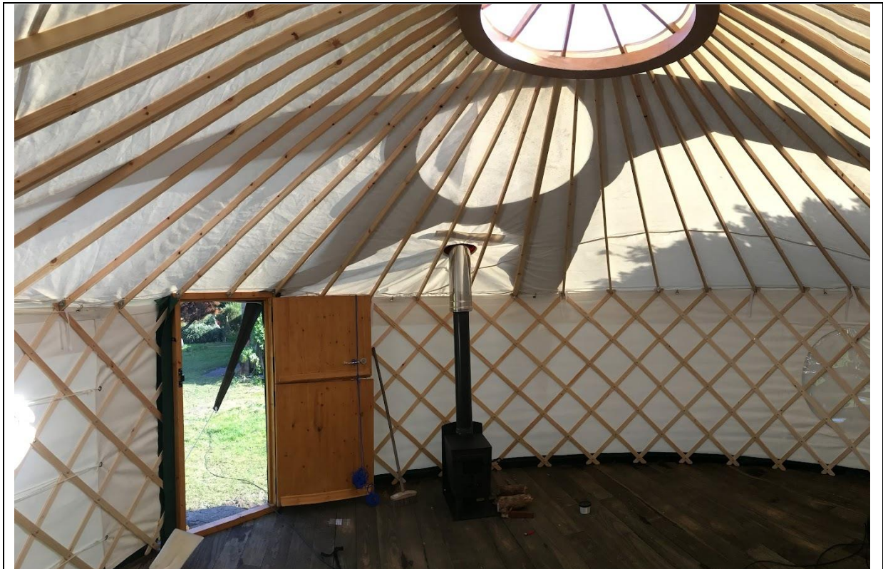
Photo 1 – showing the structure of the yurt.
