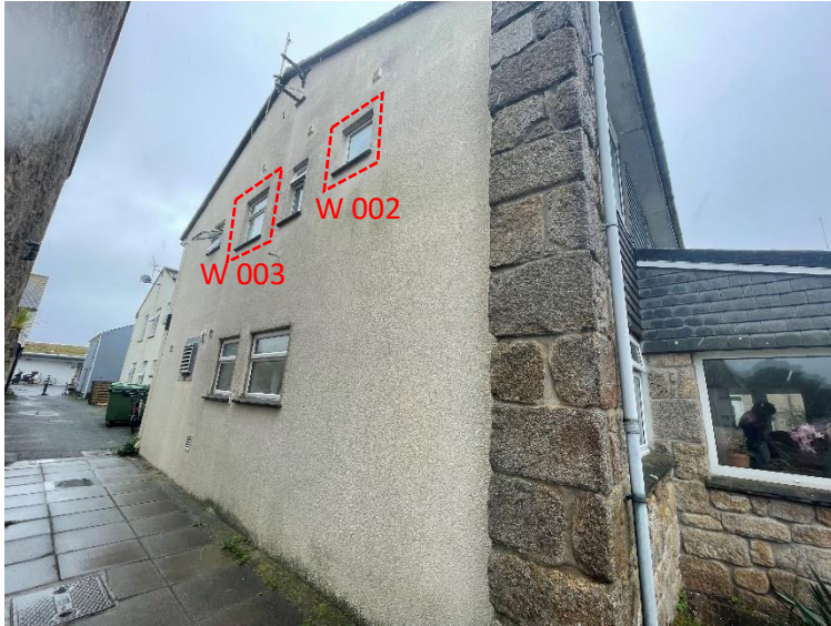
Figure 2: East Elevation – Windows to be replaced
