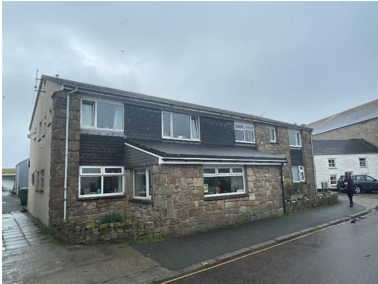
Figure 1: Front Elevation (General View)
