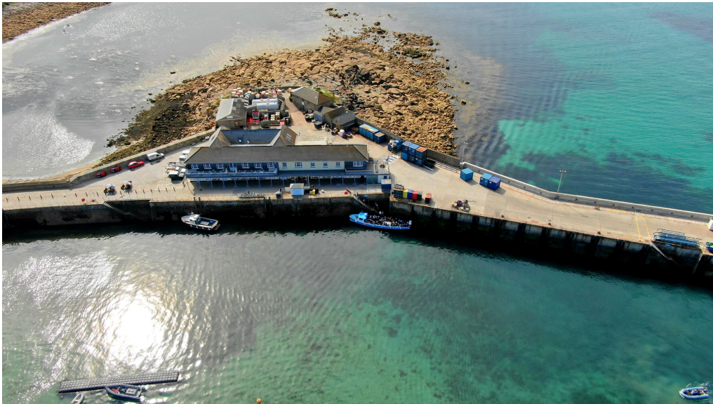
Photo 2. On the Quay. Building Photo.
