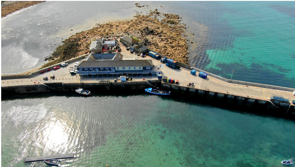
Photo 2. On the Quay. Building Photo.
