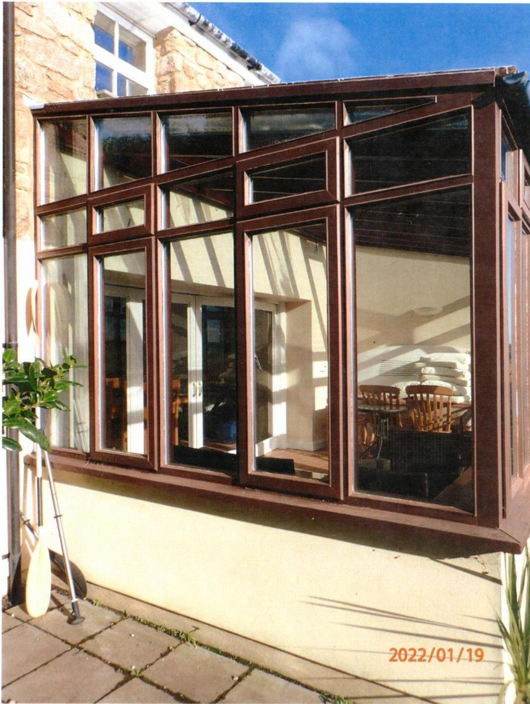
Remove middle row of glazing (windows to extend up to gutter level to match front elevation)
