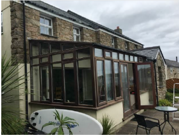
Photograph 1: Showing the conservatory attached to the main house.
