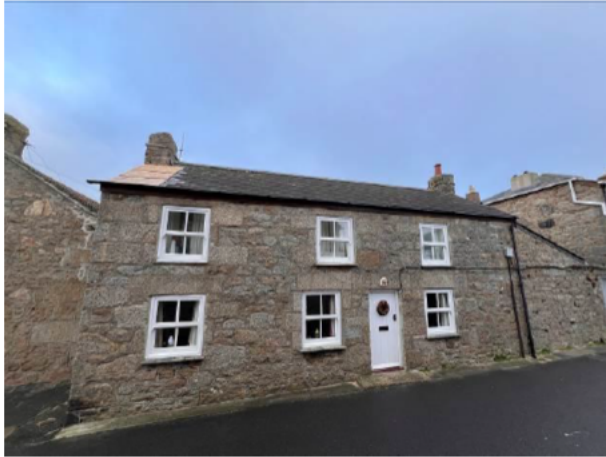
Photograph 1: Showing the property as viewed from the road to the west.
