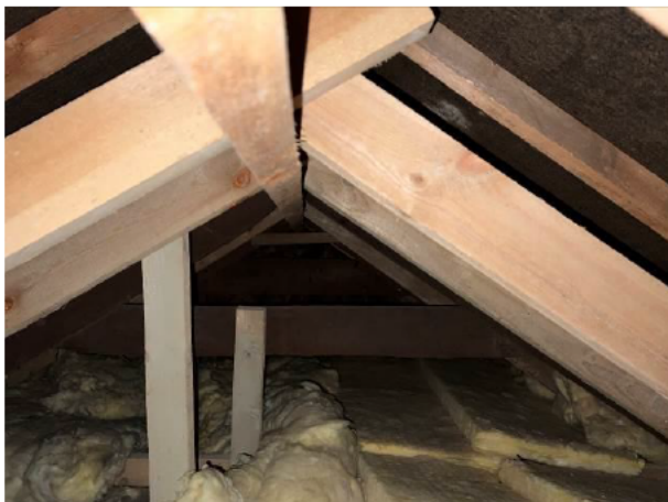
Photograph 5: Showing the interior of the loft space
