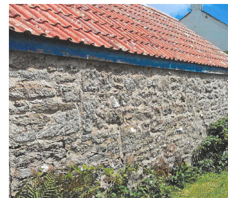
Figure: 13 External View Of Barn Wall Build-up.
