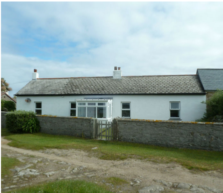
Figure: 10 Signal Rock House
