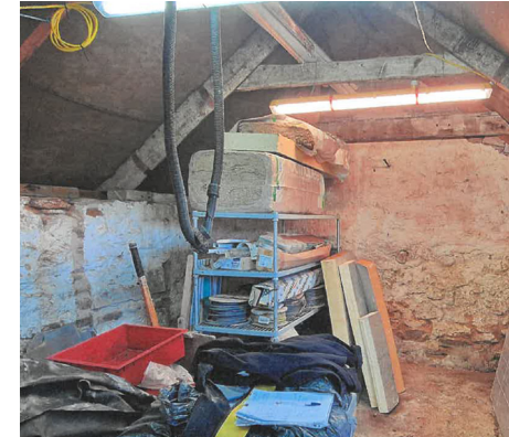
Figure: 12 Internal View Of The Roof Structure Of The Barn.
