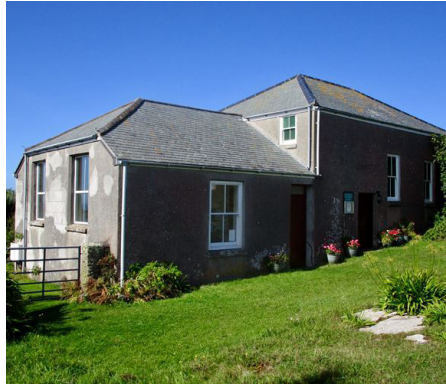
Figure: 09 Methodist Church
