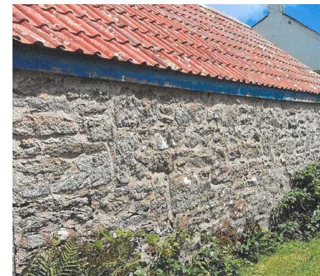
Figure: 13 External View Of Barn Wall Build-up.
