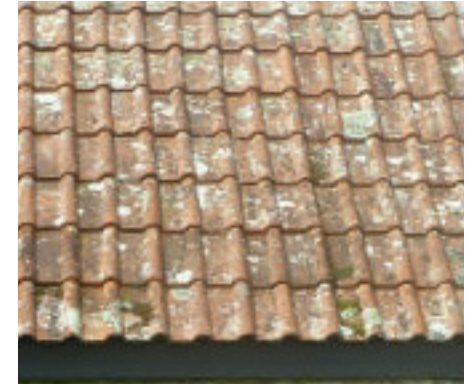
Figure: 18 Concrete Tiled Roof
