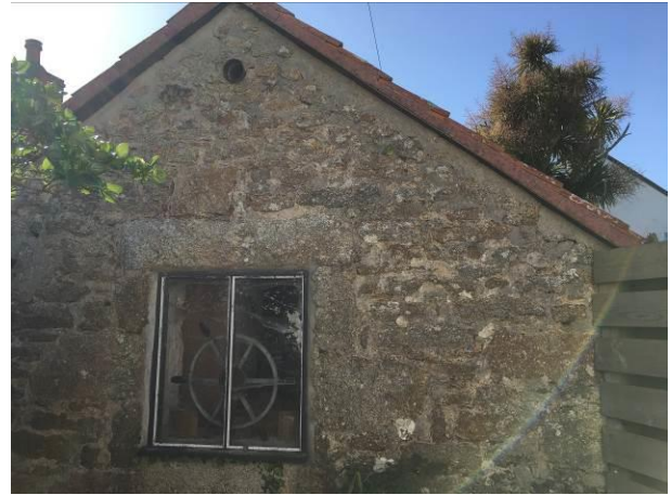
Photograph 8: Showing the south-eastern gable of the stable block.
