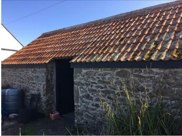
Photograph 1: Showing the north-eastern aspect of the stable block
